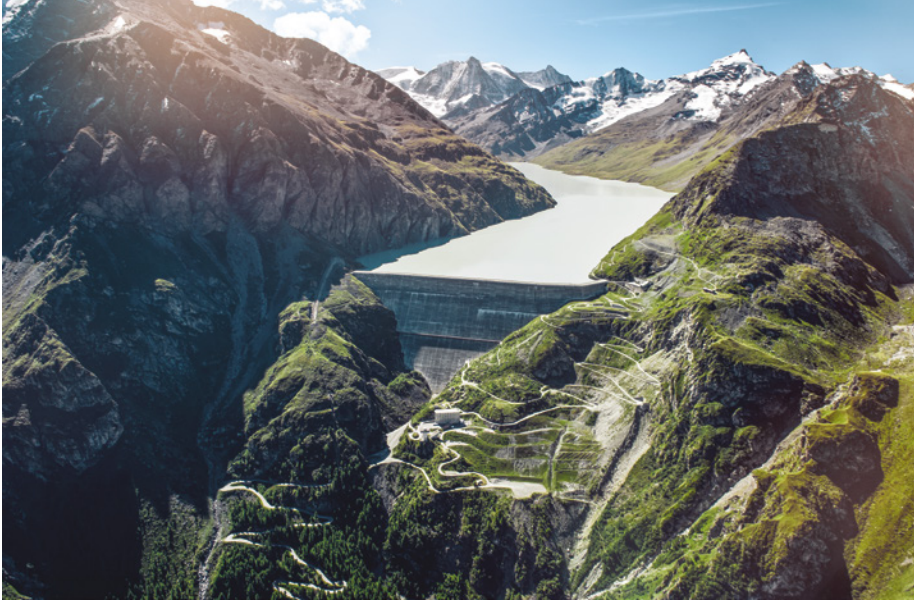
The Grande Dixence, the tallest gravity dam in the world (285 m), supplies electricity to more than half a million households.
