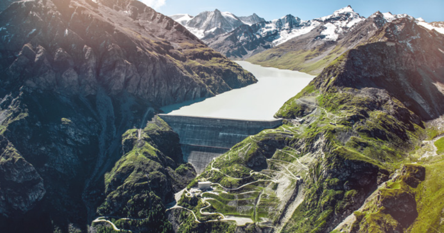
The Grande Dixence, the tallest gravity dam in the world (285 m), supplies electricity to more than half a million households.
